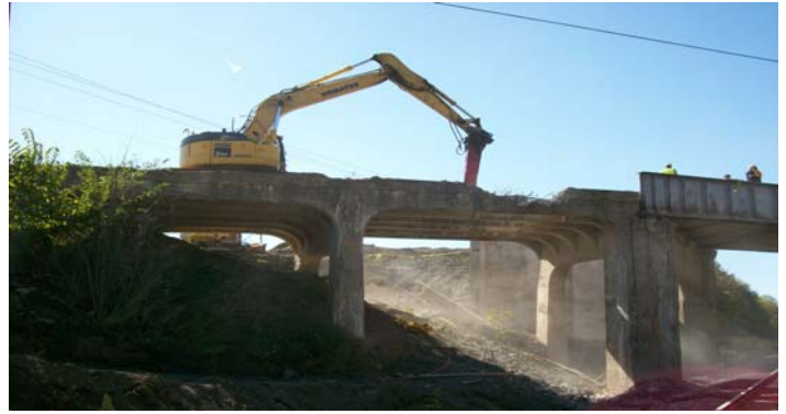
Demolition of 1925 bridge.
