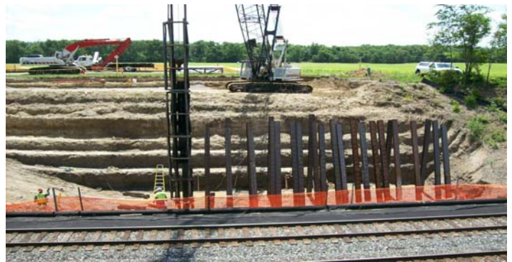
DeGraff side pile foundations.
