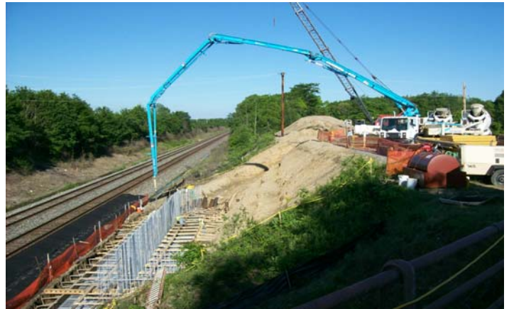
Pouring Quincy side foundation.
