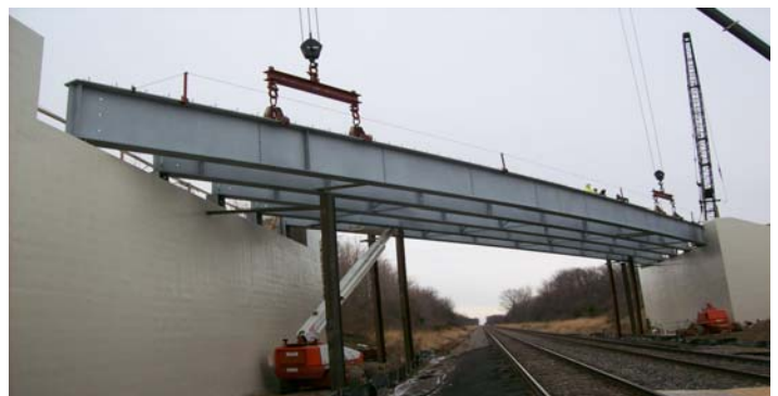
Setting girders atop new abutments.
