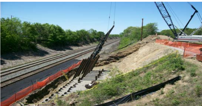
Quincy side pile foundations.
