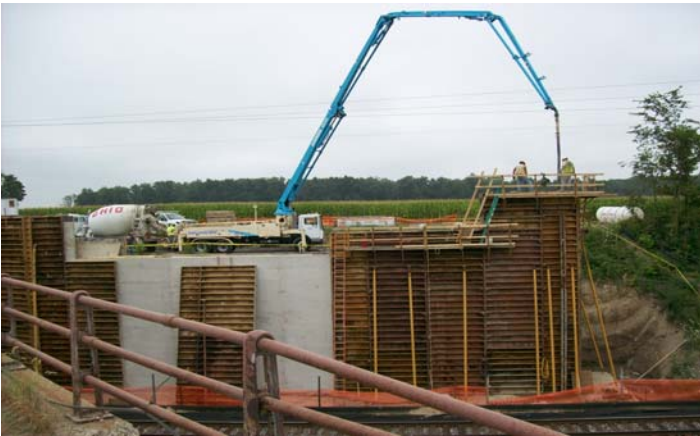
Pouring DeGraff side abutments.
